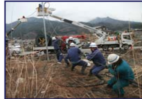
<Emergency restoration of access areas>
