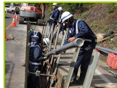
Temporary relay transmission lines
