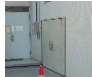
Flood prevention door
