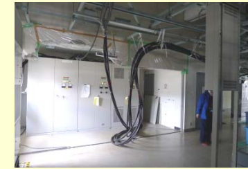
Full-fledged restoration of temporary power facilities equipment
