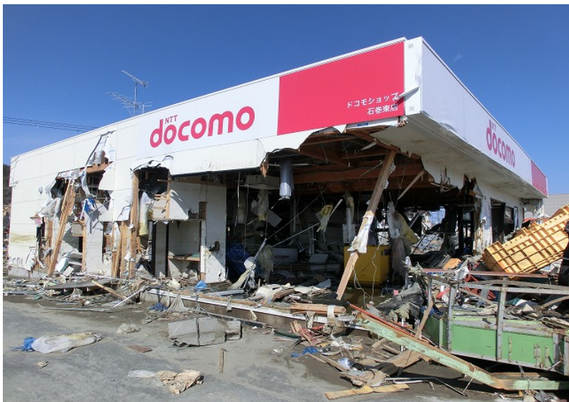
4. docomo Shop (Ishinomaki-Higashi, Miyagi)
