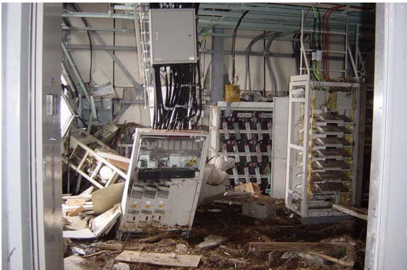
2. Transmission facility (Noda-mura, Iwate)
