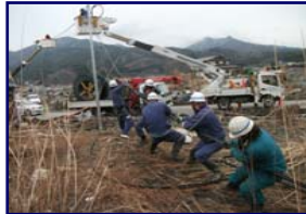
<Emergency restoration of access areas>
