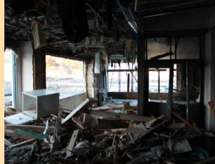
Walls were damaged and the building was filled with driftage
