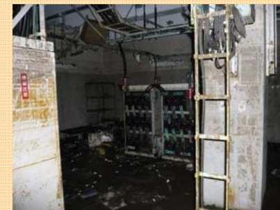
Power equipment was also greatly damaged from the flooding
