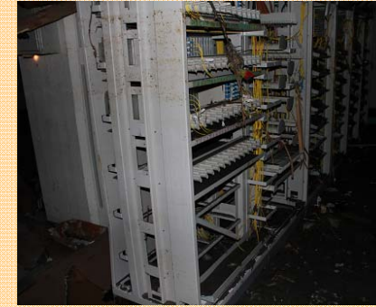
Communication equipment was also damaged by the flooding
