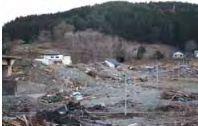
New telephone poles erected near a railway
