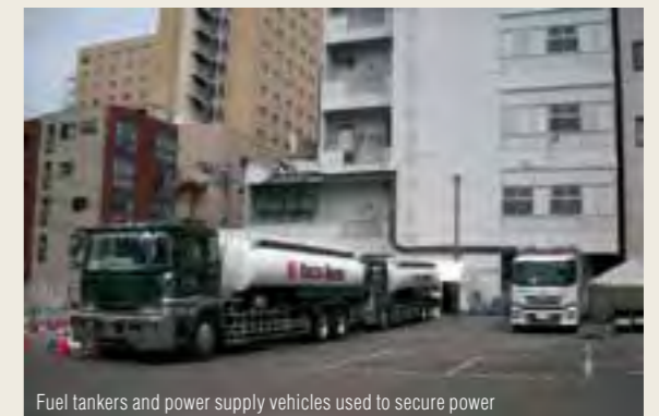
Fuel tankers and power supply vehicles used to secure power
