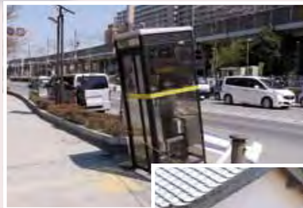
A public phone box leaning as a result of liquefaction (Urayasu City, Chiba Prefecture)
