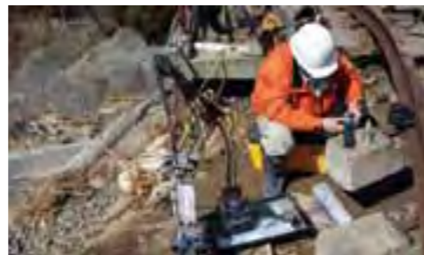
Connecting the cores of bypass cables to existing cables
