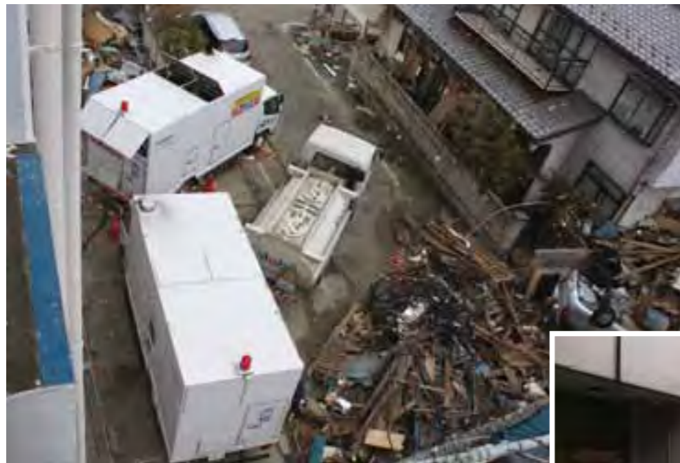
Power supply vehicle and fuel tanker keeping the Ishinomaki Kadonowaki Building running (Ishinomaki City, Miyagi Prefecture)
