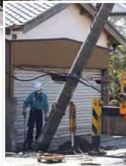
A telephone pole leaning as a result of liquefaction (Itako City, Ibaraki Prefecture)
