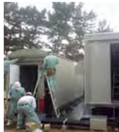
Container-like temporary exchanges slated for use elsewhere were requisitioned for installation on the site.
