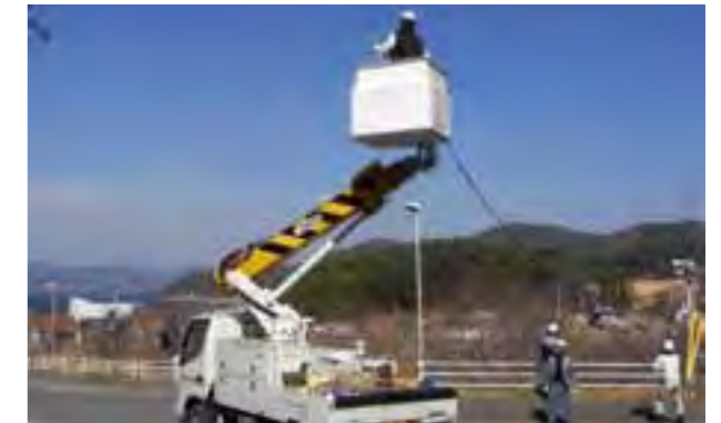
A support team from NTT West engaged in restoring access lines
