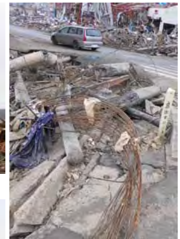
Reinforced concrete telephone poles lay shattered along every road. (Onagawa Town, Miyagi Prefecture)
