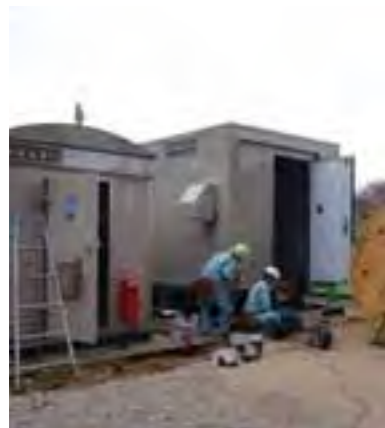
Container-like temporary exchanges slated for use elsewhere were requisitioned for installation on the site.
