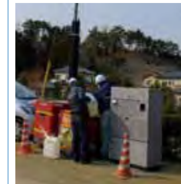
Restoring phone services by connecting subscriber cables in each area to RSBM-Fs
